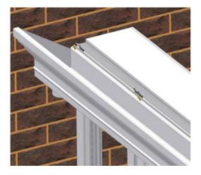
Once the guttering is in position, secure it using the Gutter Fixing Screws (C9479)
